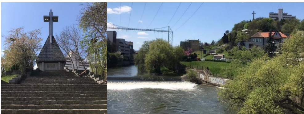
Figure 17: The Monument of the Nation's Heroes (left); Cetățuia Hill seen from the bank of the Someș river: the size of the Monument of the Nation's Heroes is observed, which competes with the Belvedere Hotel (right)
