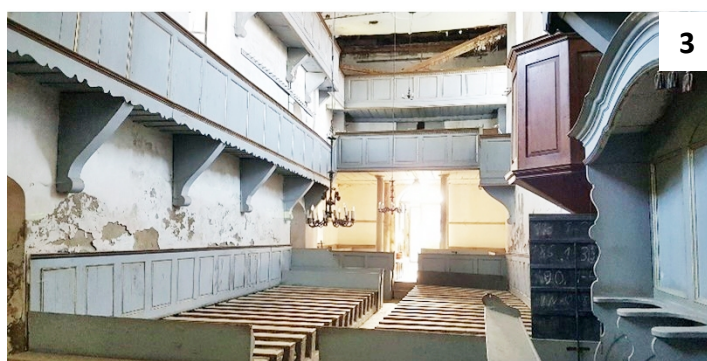
3 – Interior balconies supported by wooden consoles, 1788
