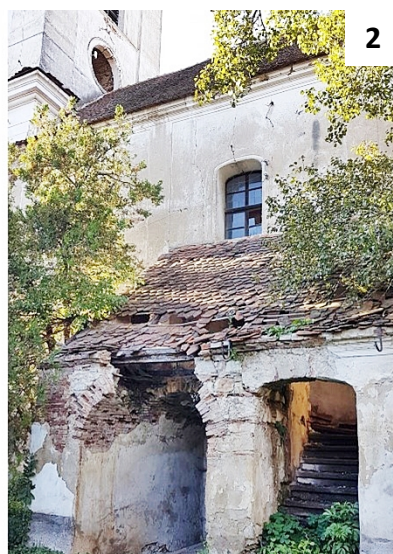
2 – Access to the balconies
